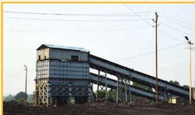
Coal Handling Plant Lingaraj
