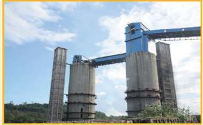
SILO under construction at Bharatpur Area
